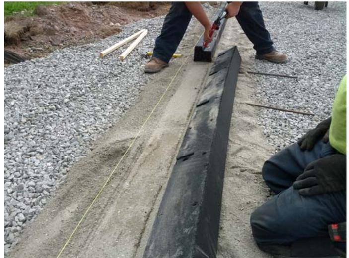
3. Once you have the correct height for the base, continue the leveling and compacting where the curb is to be placed. We usually find it a time saver that while the base work is being completed some of the crew is placing the curbs out loosely around the perimeter. Be careful not to disturb the compacted base.
