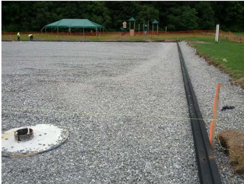
14. Using the (2 Part) Top Coat Urethane, paint all areas of the curb that will be exposed to sun light. **Two coats are required.**
