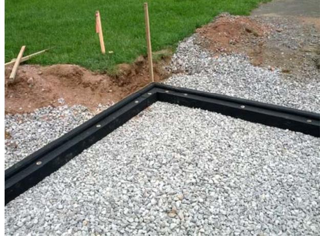
6. Using the pre drilled holes in the curb base drive the supplied 18 inch anchors into the ground. Follow the sight string line carefully, so the side of the curb is straight, not wavy. If one person places his foot (out of harm's way) on the curb, while the anchor is being installed, this will prevent the curb from moving and displacing the base.
