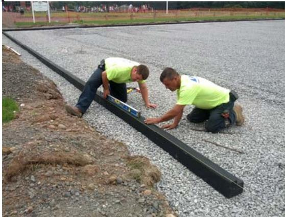
11. Once the curb is pushed tightly against the previously anchored curb, knock in the anchors.
