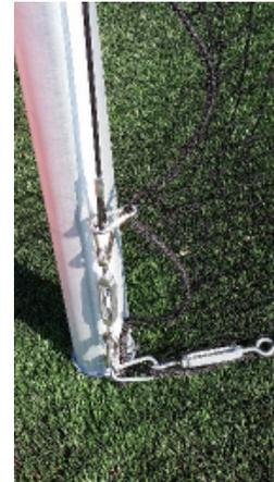
**Photo 2A, 2B & 2C** (Upper and Lower Eyebolt Connection to Looped Cable; Turnbuckle Locations)
